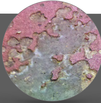
Epoxy &amp; Paint
