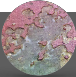
Epoxy &amp; Paint
